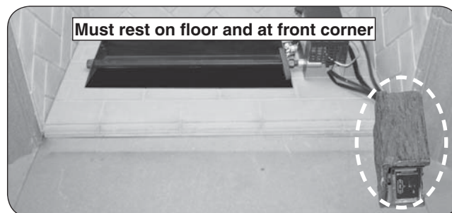
Fig. 9-3 Place heat shield
