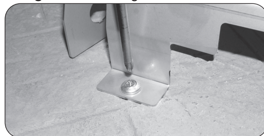
Fig. 15-2 Fastening hammer screws
