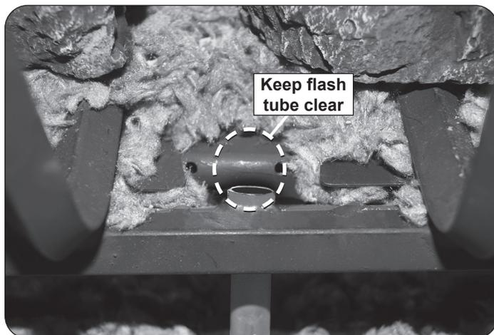
**DO NOT** place any embers on top of the flash tube to ensure proper operation. **Keep the area shown above clear at all times.**
