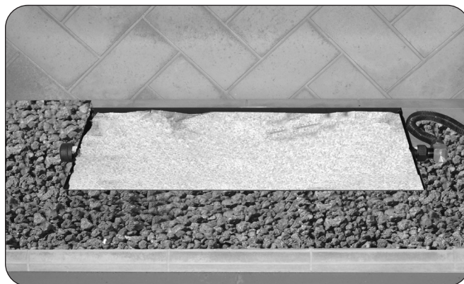
Fig. 12-1 Place sand/vermiculite
